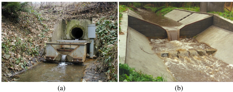
Figure 3: Gauging station for sub catchments (a) and the weir at main catchment outlet (b)
