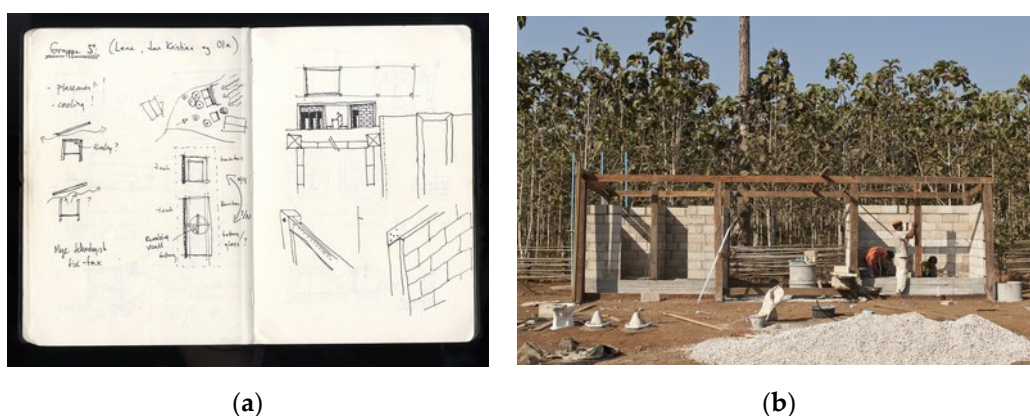
Figure 6. (a) Design on site—sketches. (b) Community building. Sketches of the designers and photo of the building process TYIN Tegnestue Architects (Andreas G. Gjertsen, Yashar Han-stad), Available online: http://www.tyinarchitects.com/downloads/ (accessed on 14 July 2021).
