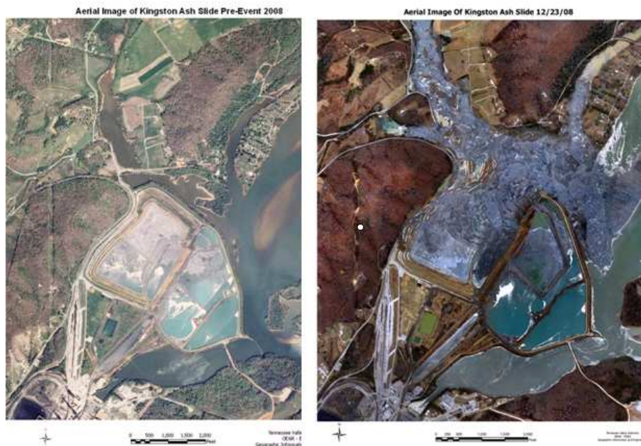
Figure 2: Gray ash hazard, USA 2008 Source: aol news, Google Earth
