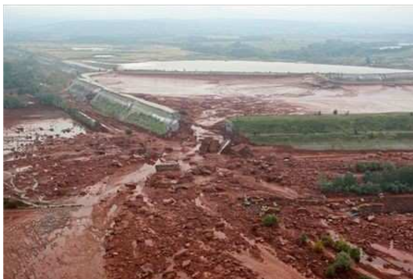
Figure 6: Picture of the flooded containment pond after the dyke broke Source: MTI
