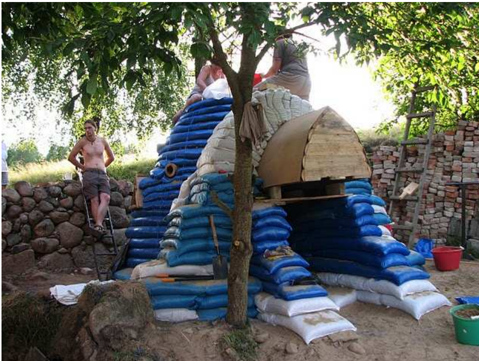
Figure 4: Sandbag shelter under construction
