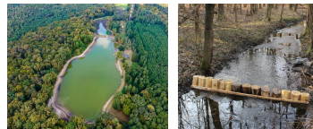
Figure 3. Reservoirs Küvölyg & a newly built log weir.
