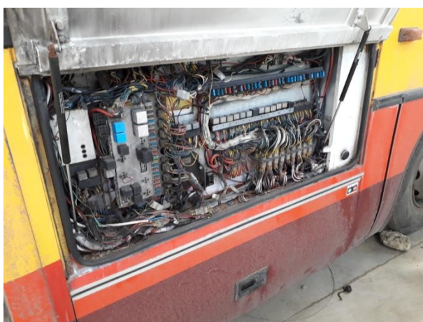
Figure 7. Main electronic control unit
