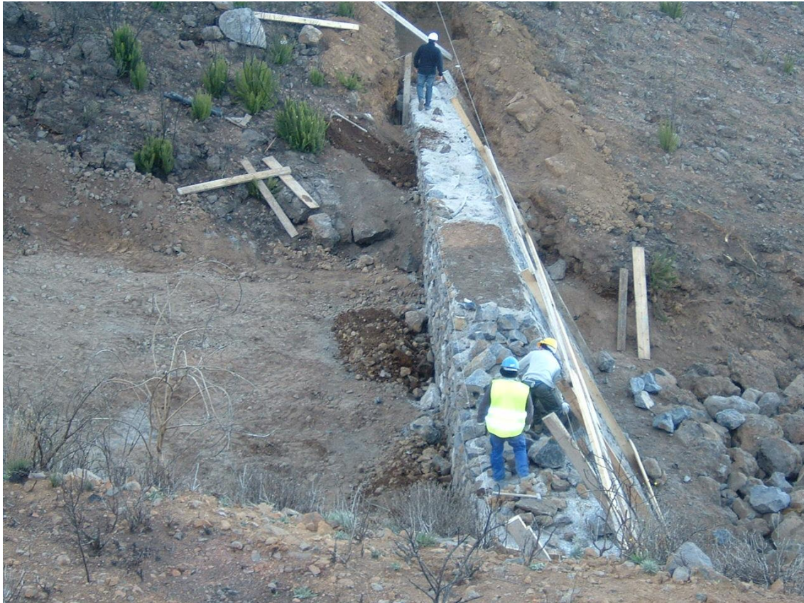
Figure 2. Construction of a sediment retention dam
