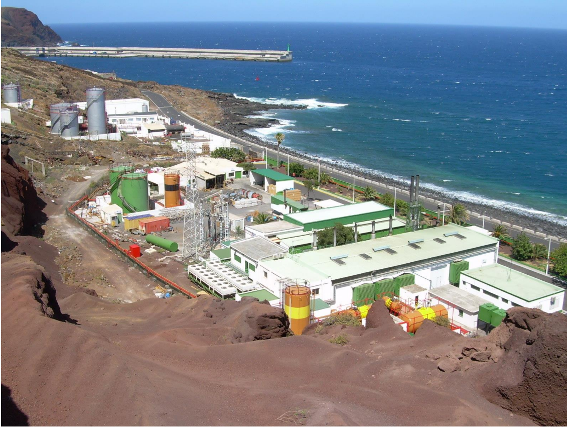
Figure 2. Diesel Electrical Power Plant on the island of El Hierro, Canary Islands
