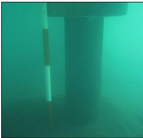
Figure 2. The wooden pile submerged in Hévíz lake.
